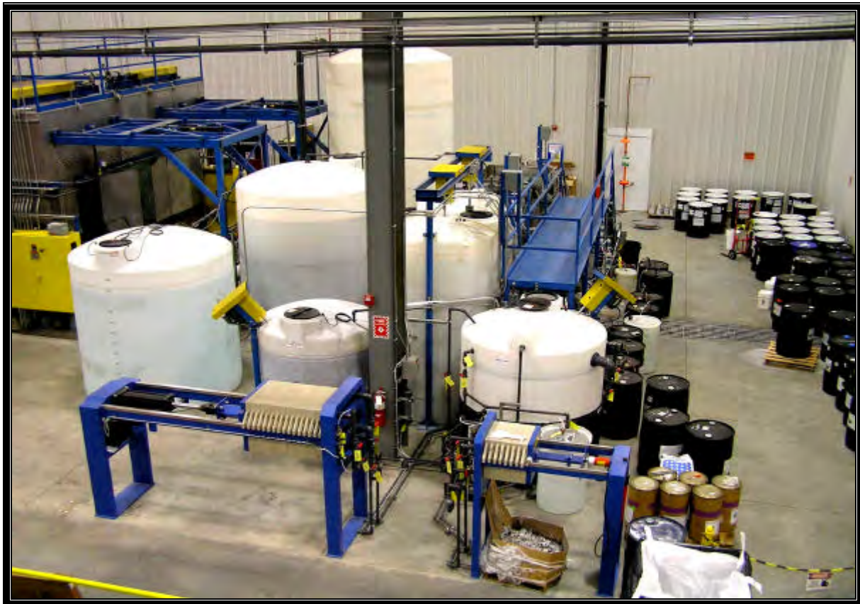
Figure 7. The wastewater treatment system handles discarded paint from all five color tanks, along with pretreatment waste.
